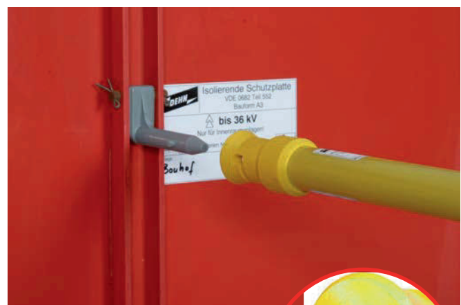
Coupling for T pin shafts
